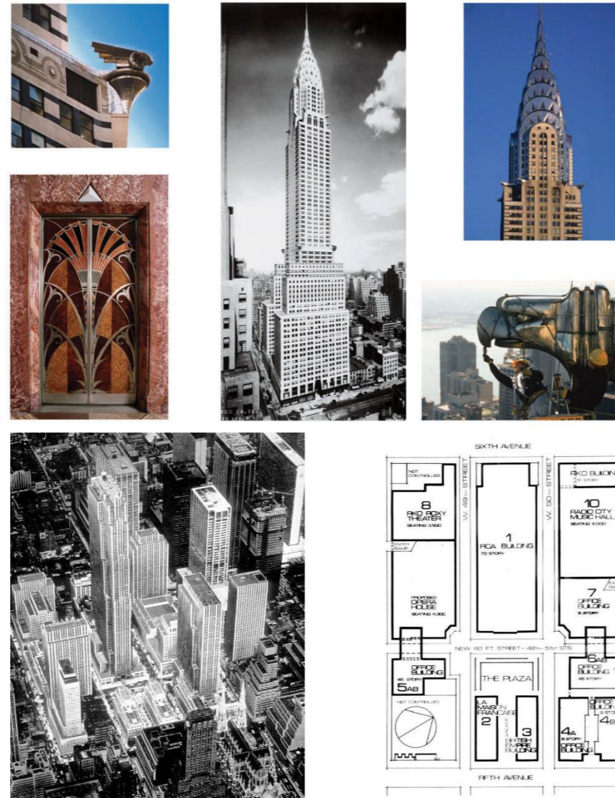
Prilog 2: Van Alen: Chrysler Building (gore); Raymond Hood & ARCH: Rockefeller Center (dolje)
