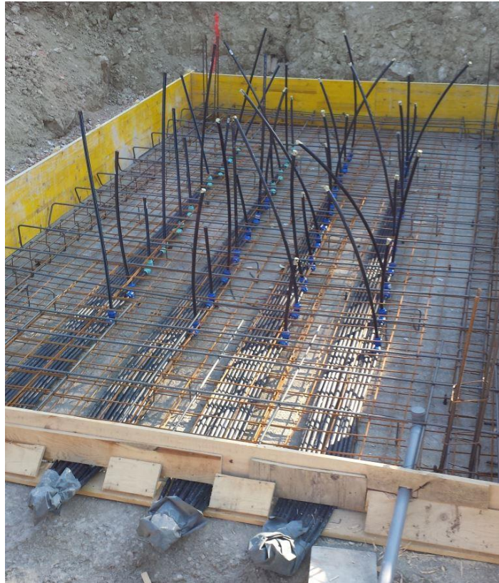
FIGURE A.19: Installation of piezometers.
