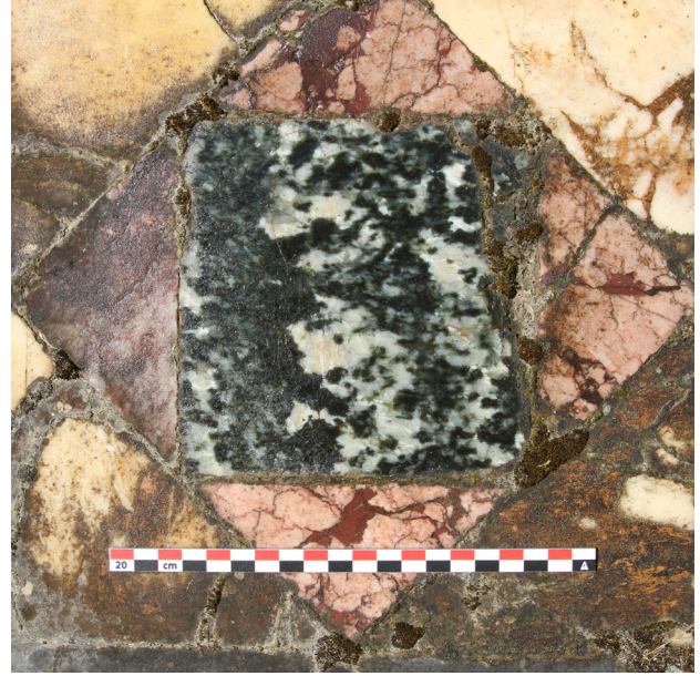
Fig. 15. Pompeii, House of M. Lucretius, tablinum (15), detail of a panel of gabbro eufotide from Egypt's Wadi Maghrabiya (photo: S. Barker)
