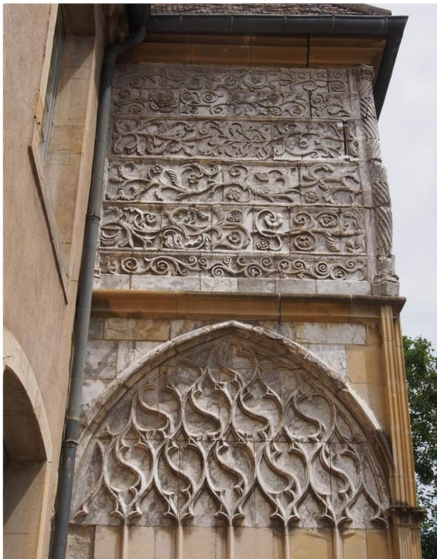
Fig. 4. Palais Jacques d'Amboise (Cluny, France), facade ornamented with alabaster sculptures dating from the early 16 th century, and restored in 1938 (photos: W. Kloppmann)
