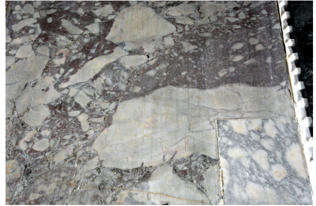
Fig. 8. Hagia Sophia, main pier, rosy breccia panel (Lydian marble?) with Phrygian marble ( pavonazzetto ) patch
