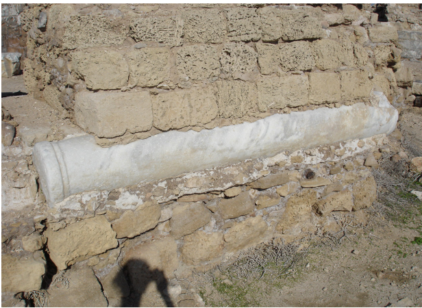
Fig. 5. Reused column as wall stabilization of the Crusader fortress
