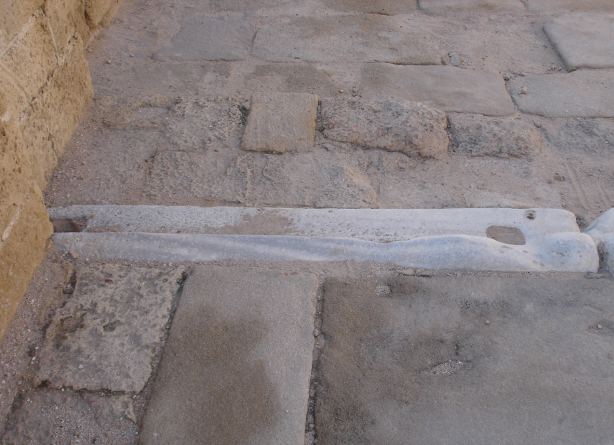
Fig. 4. Reused column as a threshold of the Crusader fortress gate
