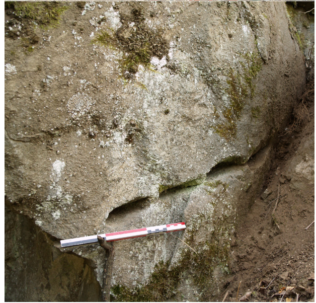
Fig. 8. Wedge holes in the quarry and on a block from the fortification core (photo: B. Djurić)
