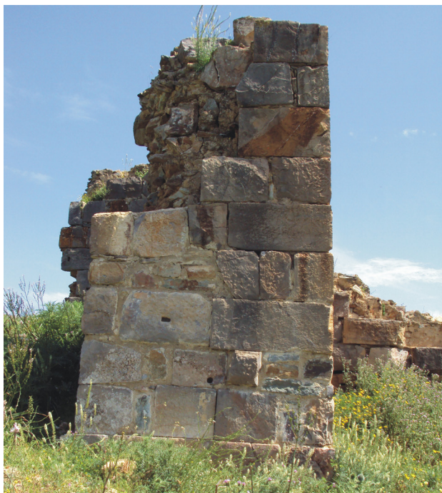
Fig. 12. Green schist squared blocks used to build a Byzantine tower (photo: A. Younès)
