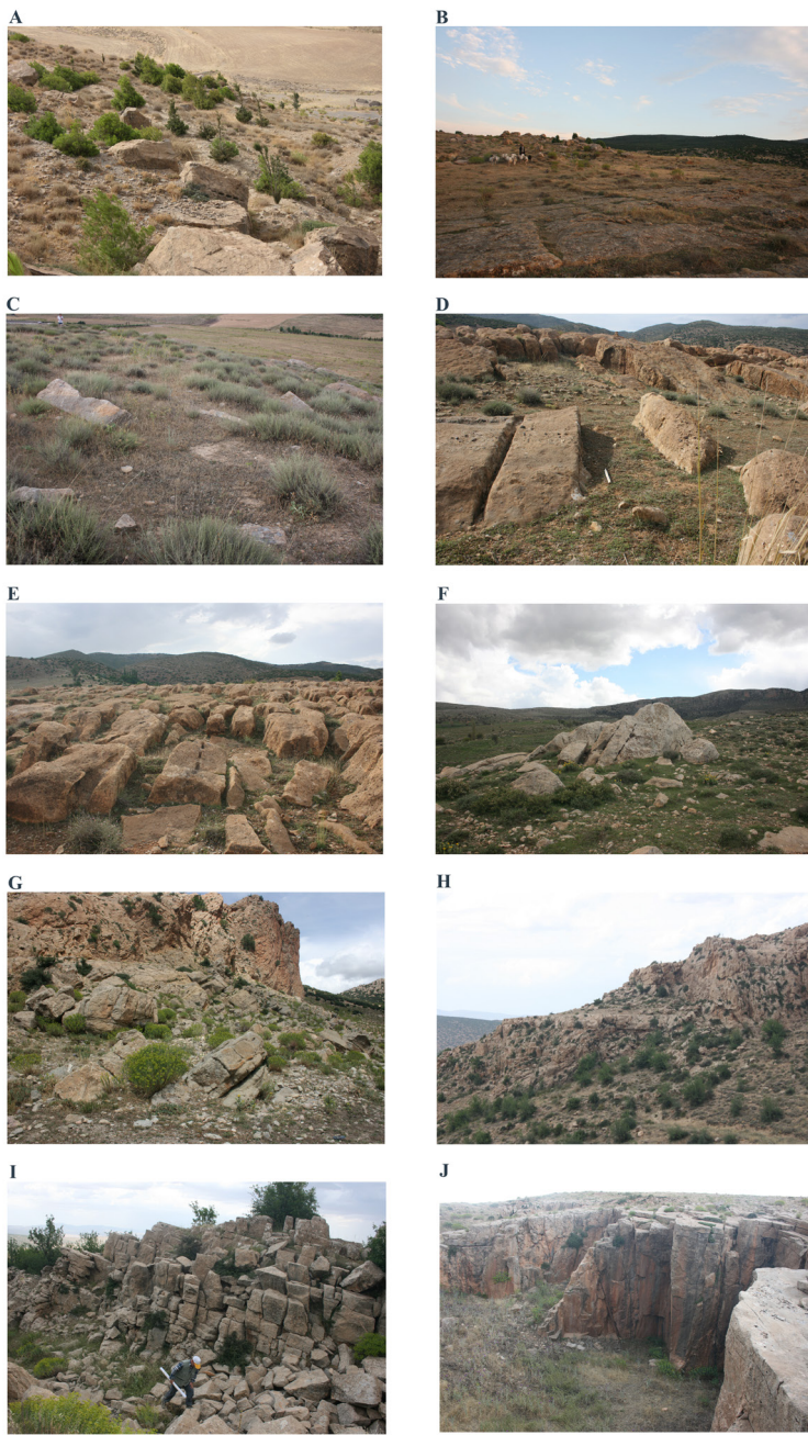
Fig. 6. General view of the limestone quarries, extraction sites and outcrops around Thamugadi. A: Djebel Afia quarries; B: Ain Drinn outcrops and exploitations; C: Lambese exploitations; D: Opencast quarries of Taouint Abderahmane; E: Eastern extraction site in Taouint Abderahmane (red marmoreal sandstone); F: Medjeba opencast quarries; G: Berbaga outcrops; H: Ain Cherchar outcrops; I: North-western part of Lardham opencast quarries; J: Elghar Nithviren limestone quarries (Site 2)
