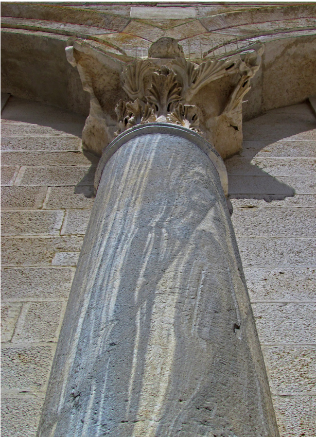
Fig. 3. Peristyle, west colonnade, a Proconnesian marble column. Toolmarks are still visible (photo: G. Nikšić)
