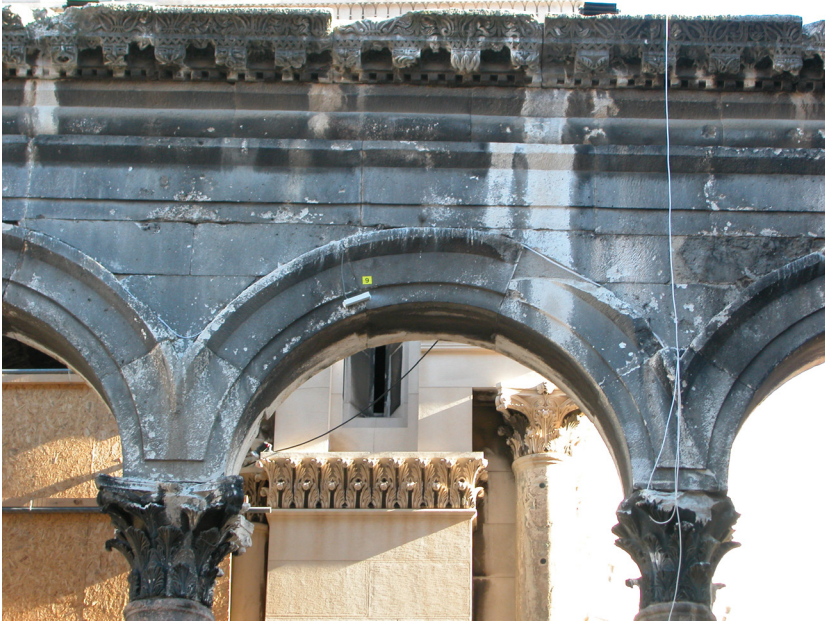
Fig. 7. Peristyle, east colonnade, detail before restoration (photo: G. Nikšić)
