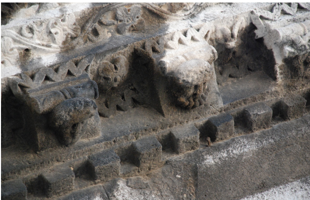
Fig. 9. Peristyle, cornice of the Prothyron gable, detail before restoration (photo: Croatian Conservation Institute)
