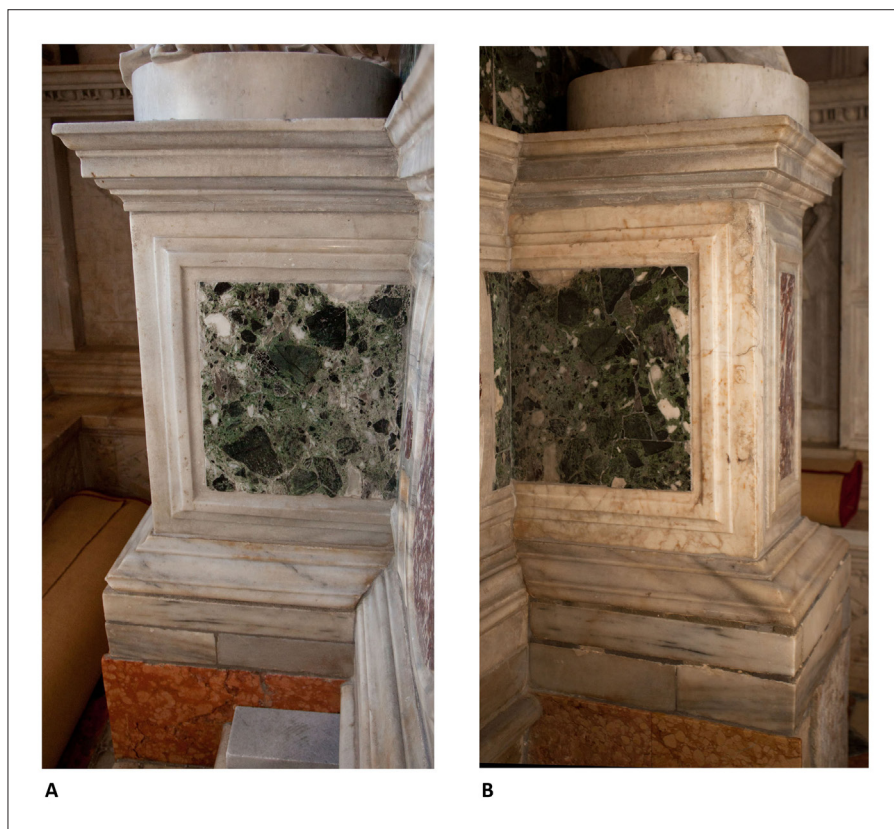
Fig. 8. Side wings of the altar: A. Western wing; B. Eastern wing (photo: Z. Sunko)
