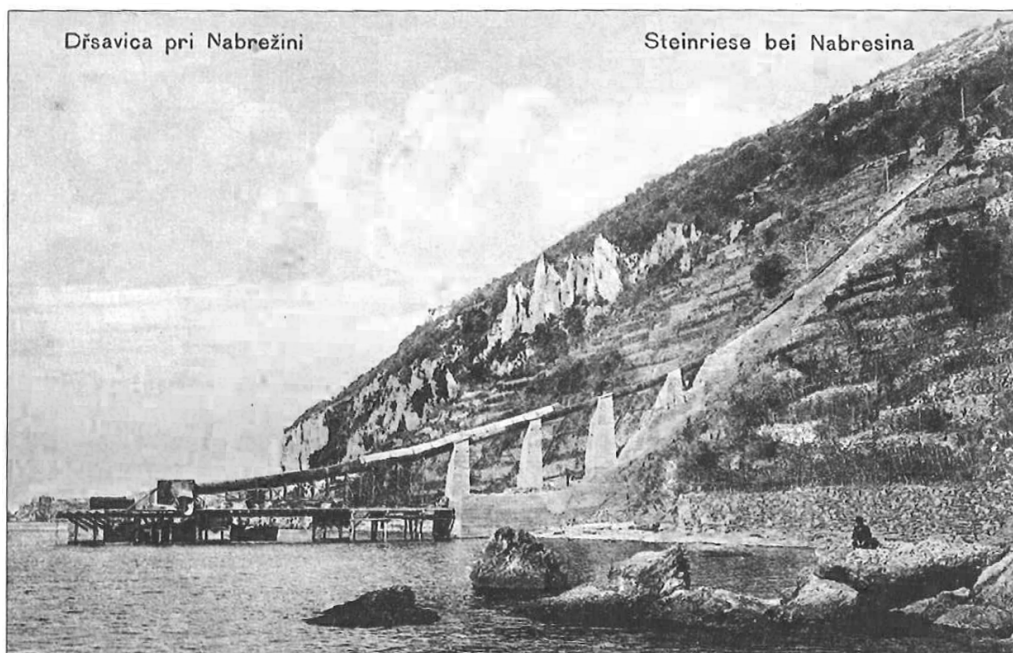
Fig. 6. A slide used at the beginning of the 20 th century to move stone chips and blocks from the quarries to the sea (from: FLEGO, RUPEL, ZUPANČIČ 2001)
