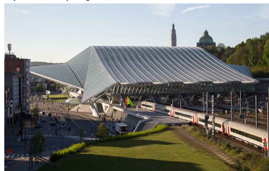
Liege-Guillemins station, Santiago Calatrava, Liege, Belgija
