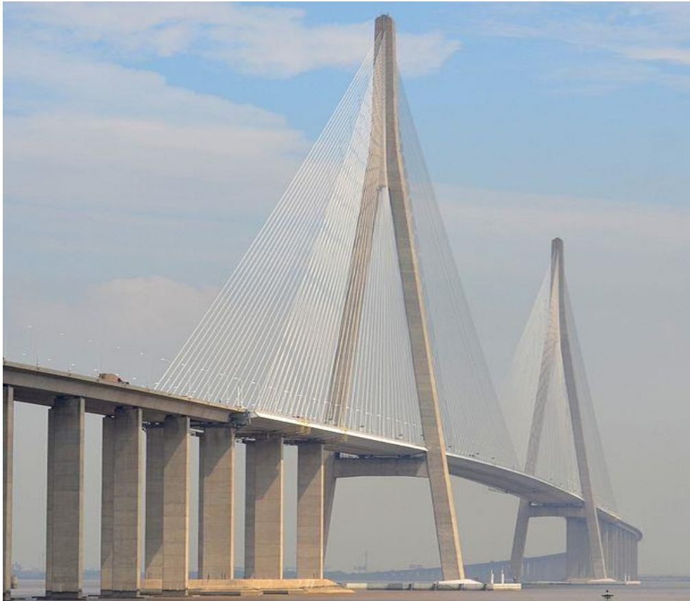
Figure 2.6 – Sutong Bridge (Wikipedia, 2015)
