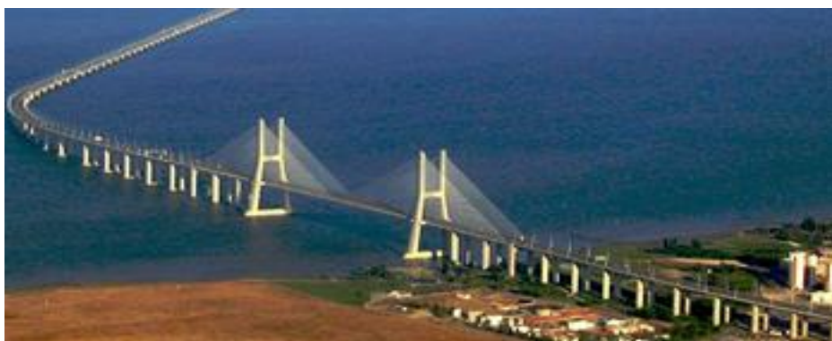
Figure 2.9 – Vasco da Gama Bridge ( http://www.thelisbnconnection.com/ , 2015)
