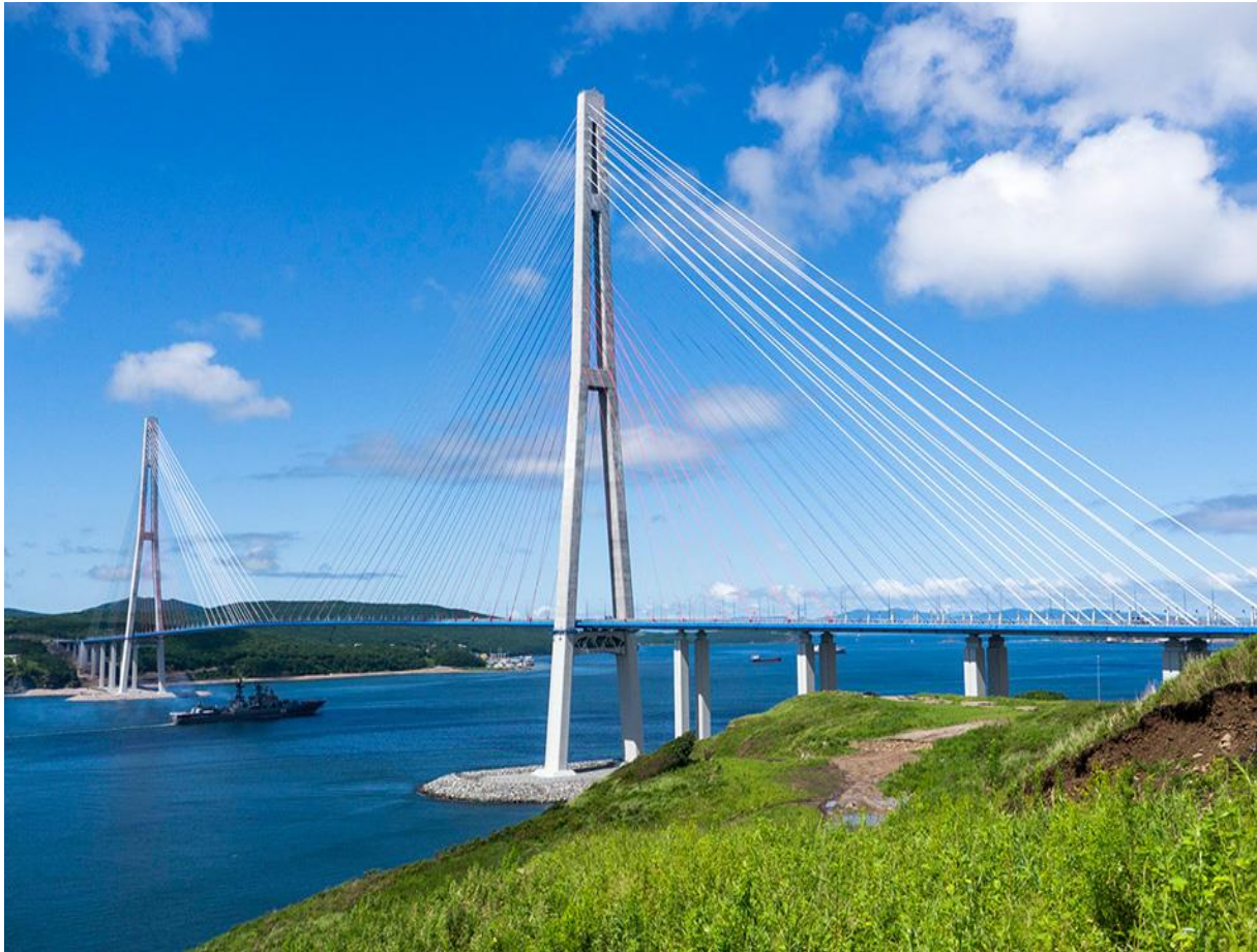
Figure 2.7 – Russky Bridge ( http://rusbridge.net/ , 2015)
