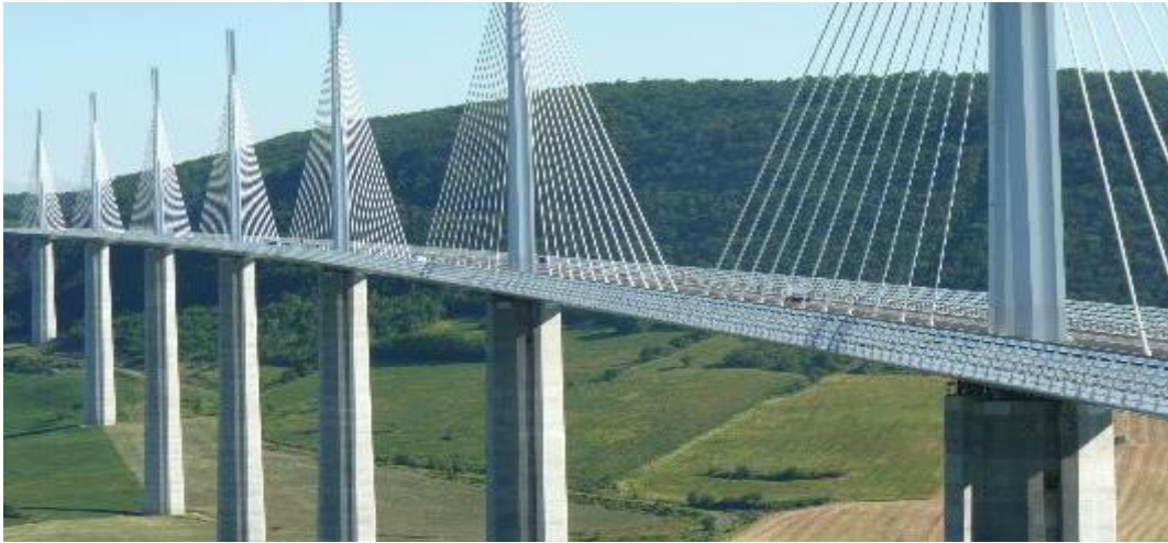
Figure 2.12- Viaduct de Millau ( http://circuitosvip.blogspot.pt/2015/01/viaduto-de-millau-franca.html , 2015)
