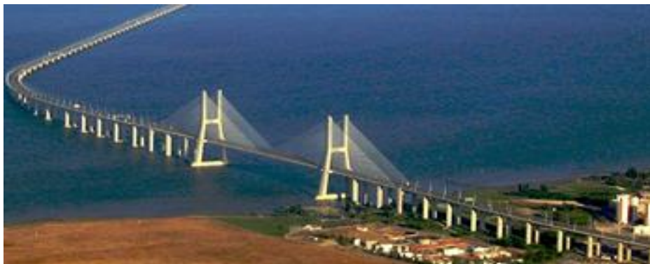
Figure 2.9 – Vasco da Gama Bridge ( http://www.thelisbonconnection.com/ , 2015)
