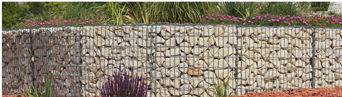
Reciklirani kamen, gabioni ,izvor: https://www.mainlandaggregates.co.uk/quarried-aggregates/quarried-gabion-stone.html
