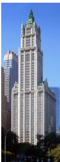
Slika 1.2.1.4 Woolworth Building, New York, 1930.
