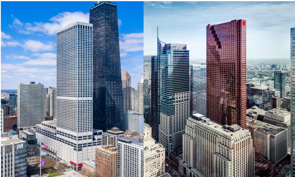
Slika 1. Water Tower Place, Chicago [3]
