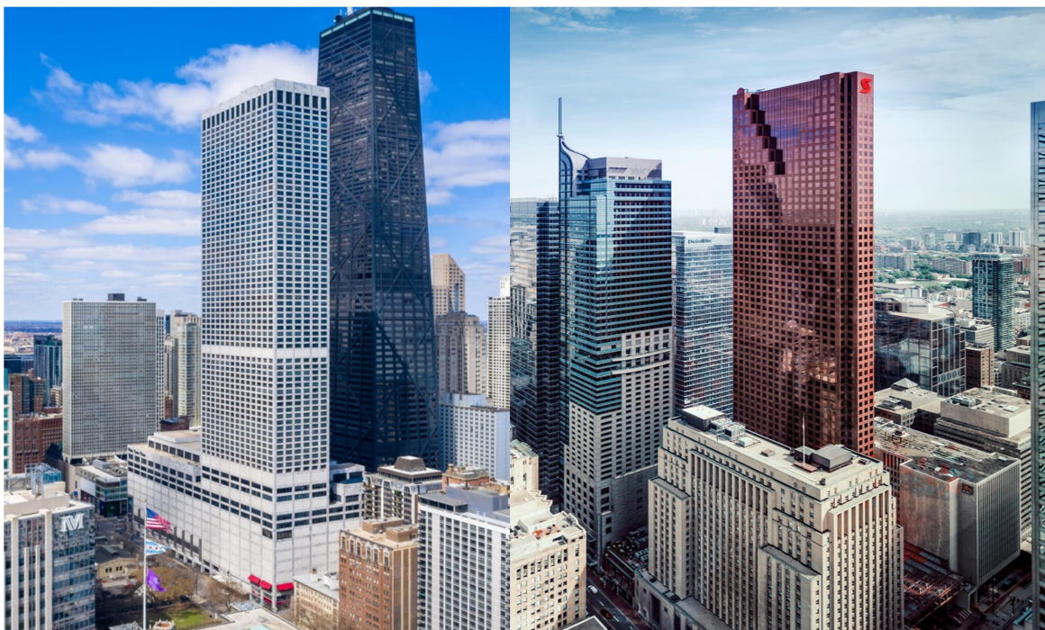
Slika 1. Water Tower Place, Chicago [3]
