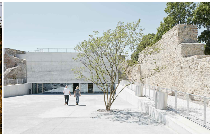
New Gallery and Casemates / Bevk Perović arhitekti
