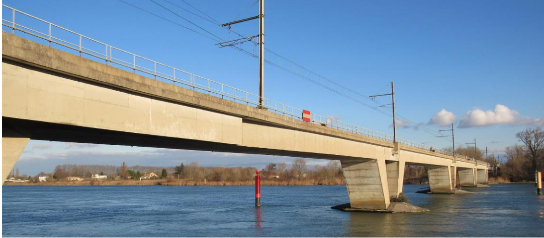
Figure 12. La Voulte railway bridge
