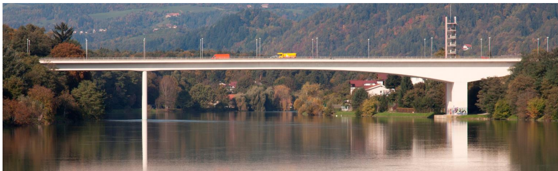
Figure 22. Carinthia Bridge in Maribor
