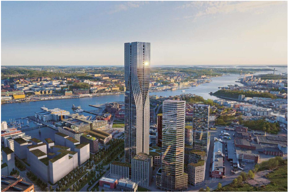
Figure 1.1 Karla tower in Gothenburg, Sweden [6]
