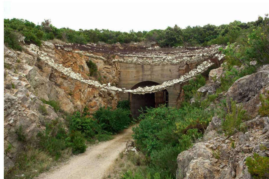
Podzemni tunel, Stupišće
