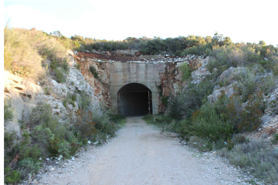
Ulaz u tunel
