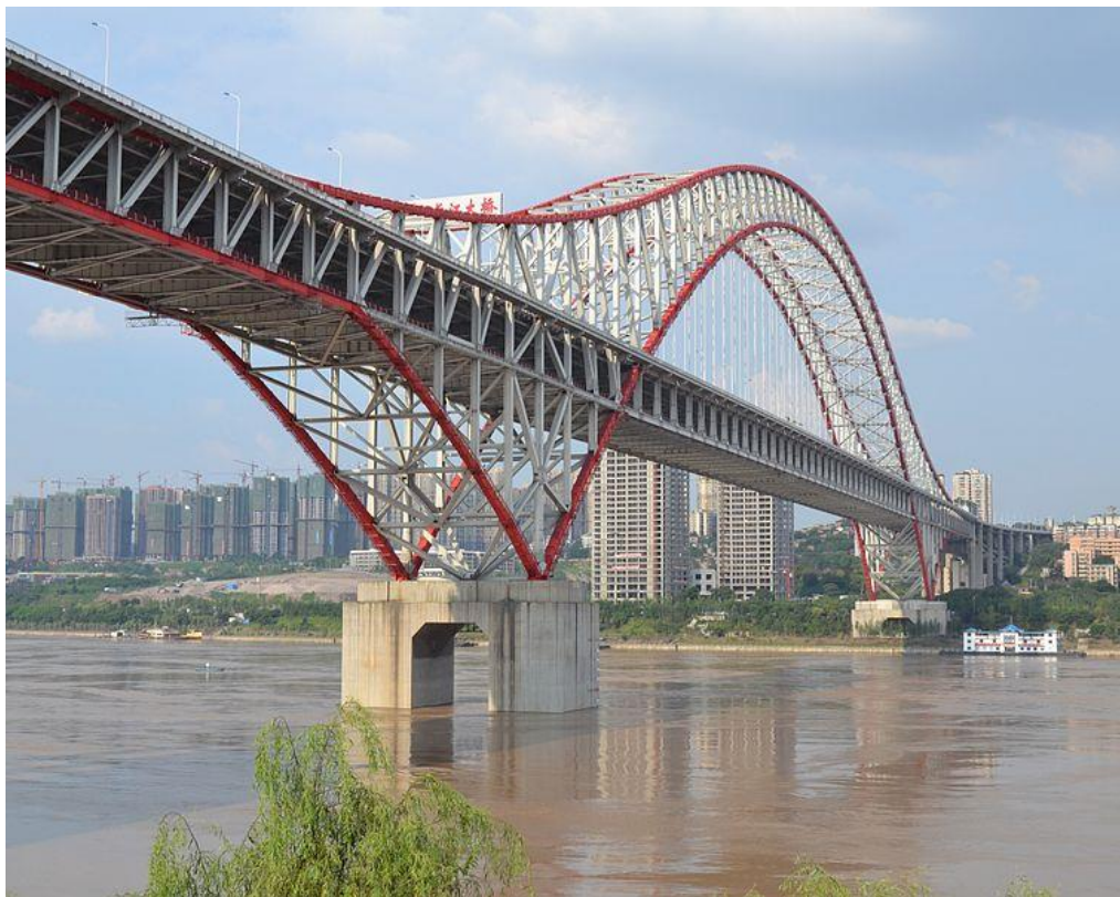
Slika 1.1.2. Chaotianmen Yangtze River Bridge
