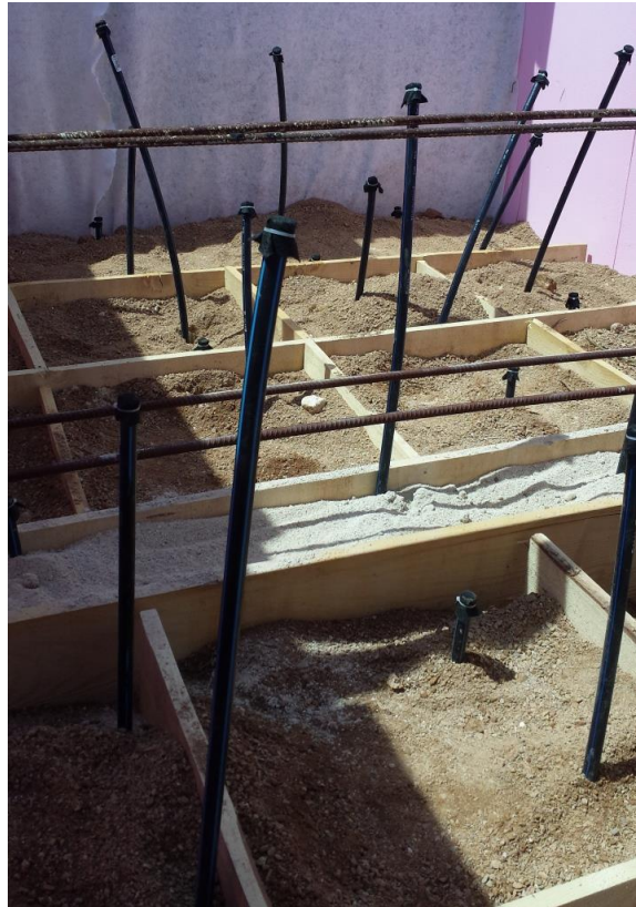
FIGURE A.5: Filling the material.
