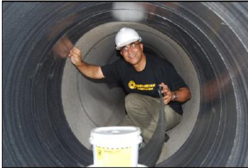
Slika 35. Spiral wound plastic liners [11]
