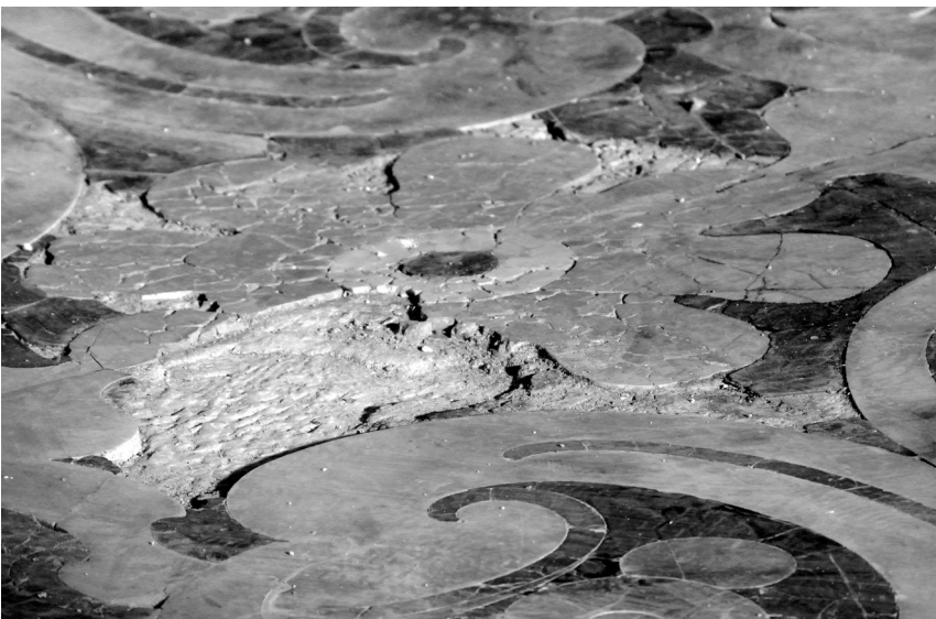
Fig. 5. Pavement of the high altar: some decay phenomena involve the marble slabs
