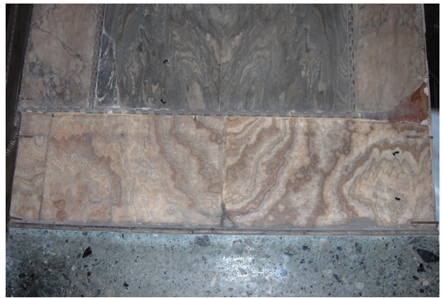
Fig. 4. Hagia Sophia, nave pier, alabastro fiorito (from Hierapolis?); above, Carystos marble ( cipollino ); below, Atrax marble ( verde antico )
