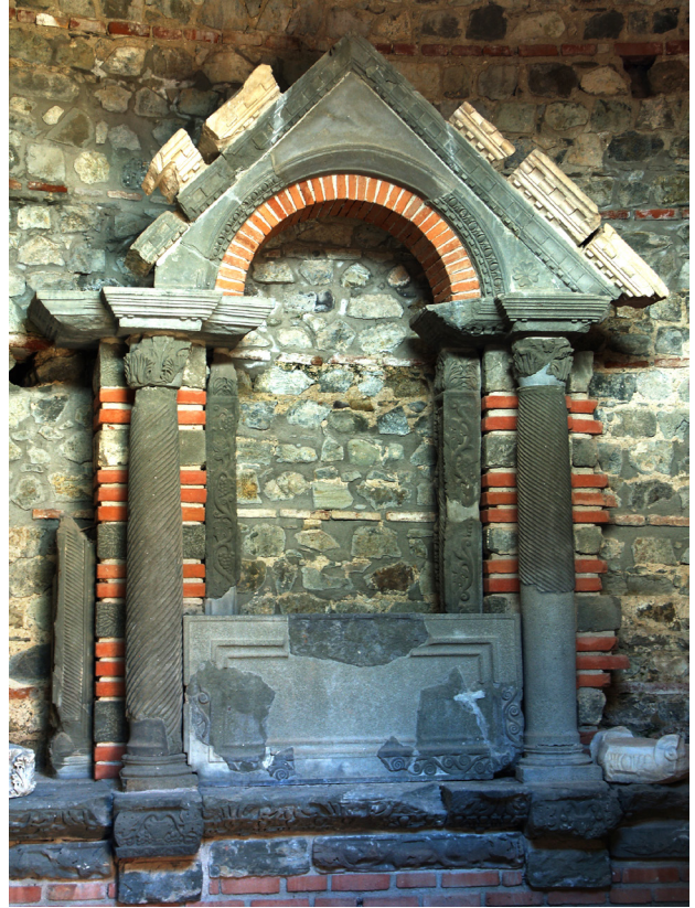
Fig. 5. Architectural elements of volcanoclastic sandstone above the gateways (photo: B. Djurić)
