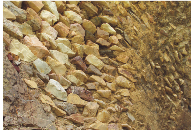
Fig. 11a. Green schist and antique yellow rubble stones used to build the cavea substructions in the Roman theatre (photo: A. Younès)
