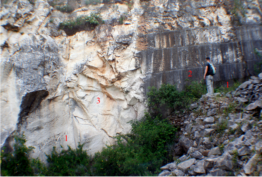
Fig. 6. Traces of a quarry on the north-eastern part of Sutvara Island with various quarrying techniques (photo: M. Parica)
