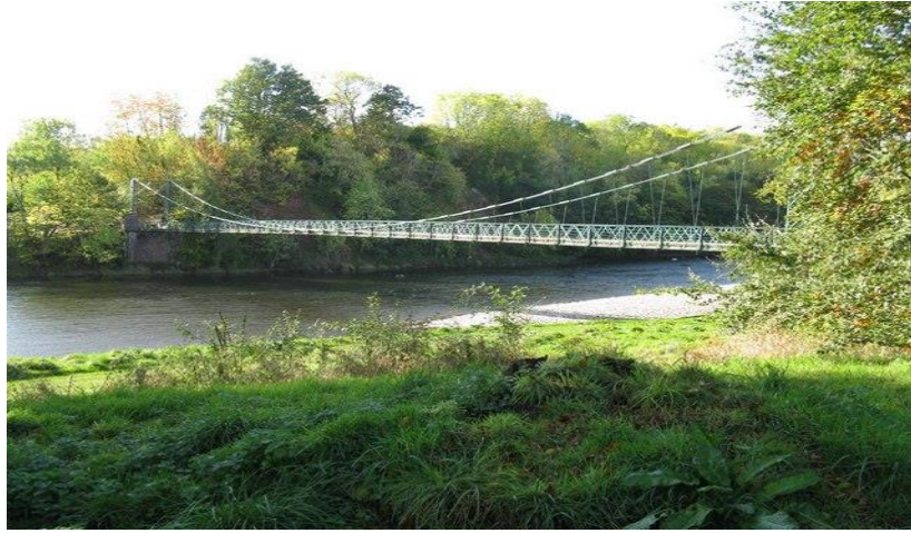
Figure 2.1 –Bridge over the Tweed river (Wikipedia, 2015)
