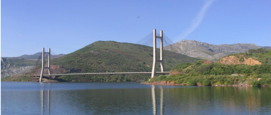
Figure 2.10 – Barrios De Luna Bridge ( http://www.arqueologiaypatrimonioindustrial.com/2007_07_01_archive.html , 2015)
