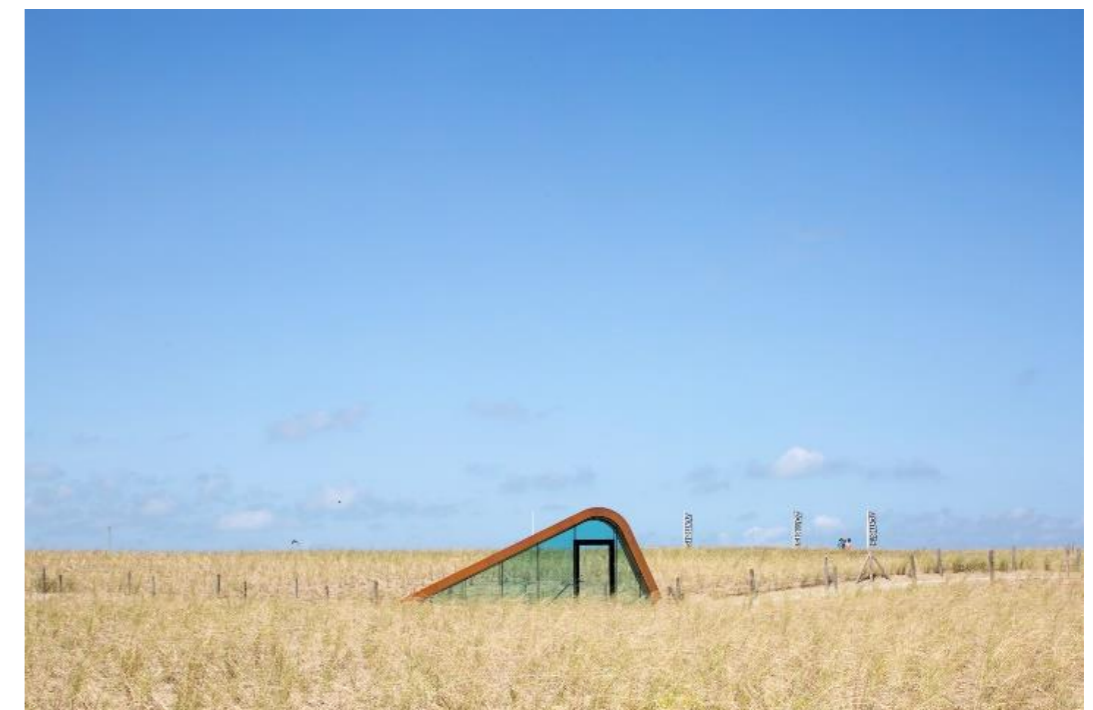
Underground parking - Royal HaskoningDHV, Nizozemska, 2016
