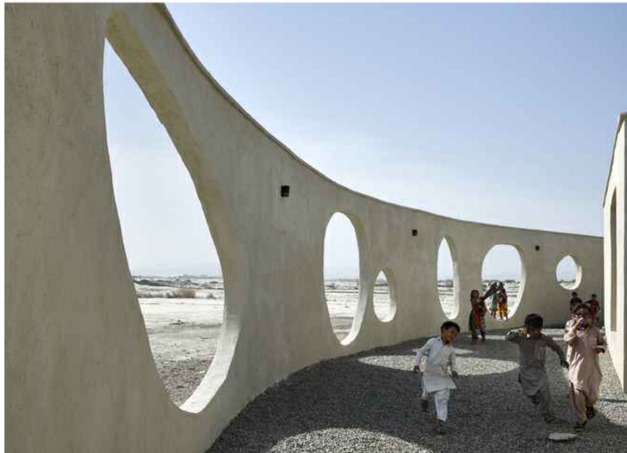
Daaz Office / Jadgal Elementary School / Iran
