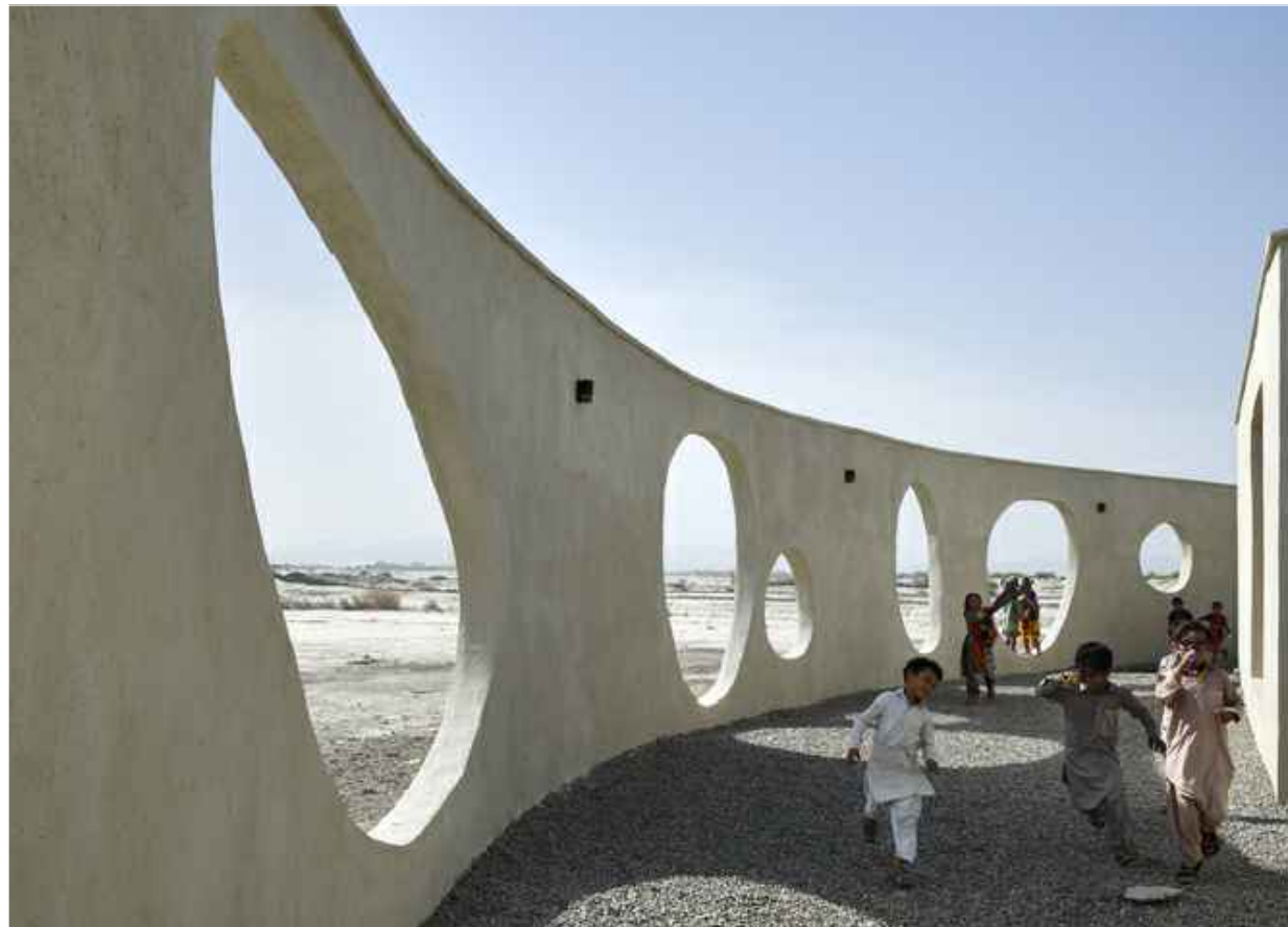
Daaz Office / Jadgal Elementary School / Iran
