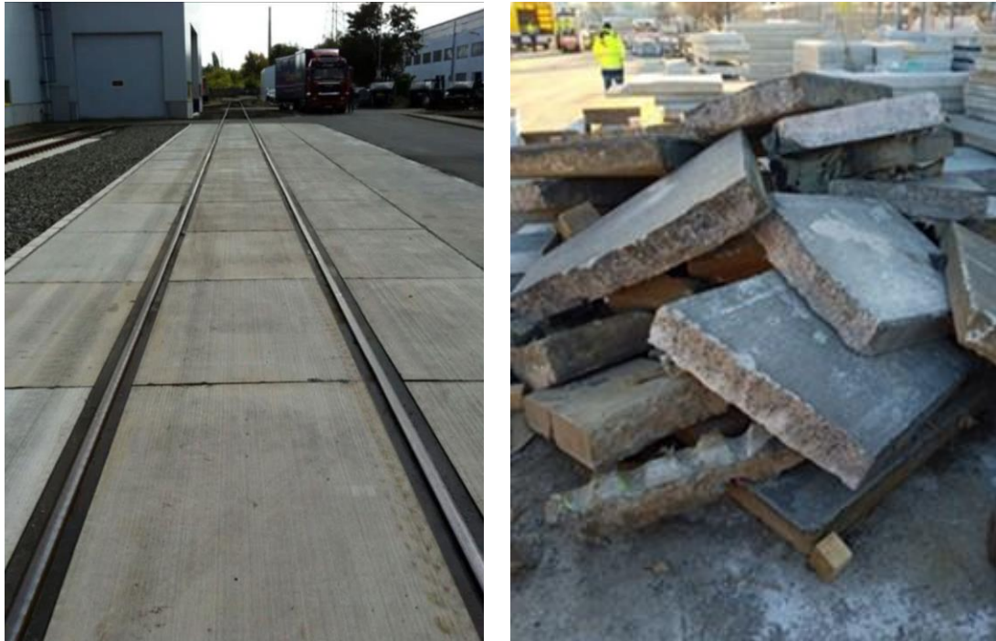
Fig. 21. On the left are panels in the usage phase in the tramway infrastructure, and on the right are the same panels after deconstruction ready for recycling
