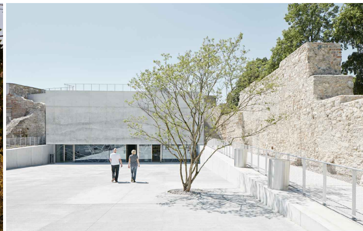
New Gallery and Casemates / Bevk Perović arhitekti
