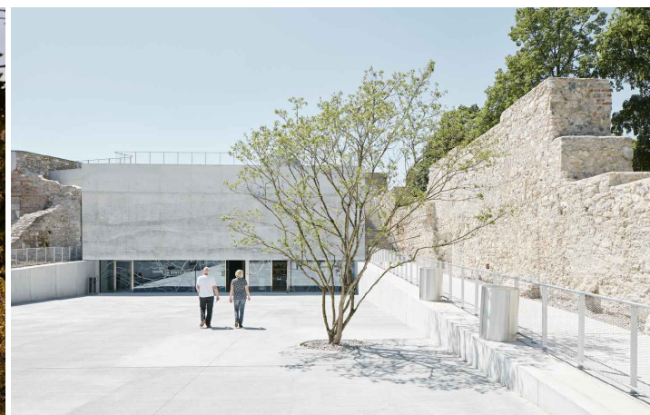
New Gallery and Casemates / Bevk Perović arhitekti
