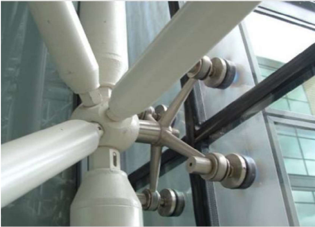
Figure 2.5 – Bolted connections [1]
