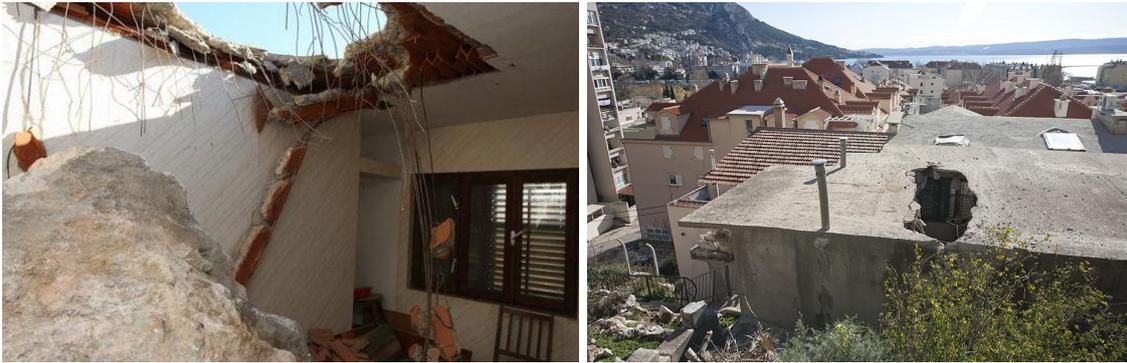
**Figure 1.3:** Severe damage of houses is caused by rock falls: Omiš, January 2012.
