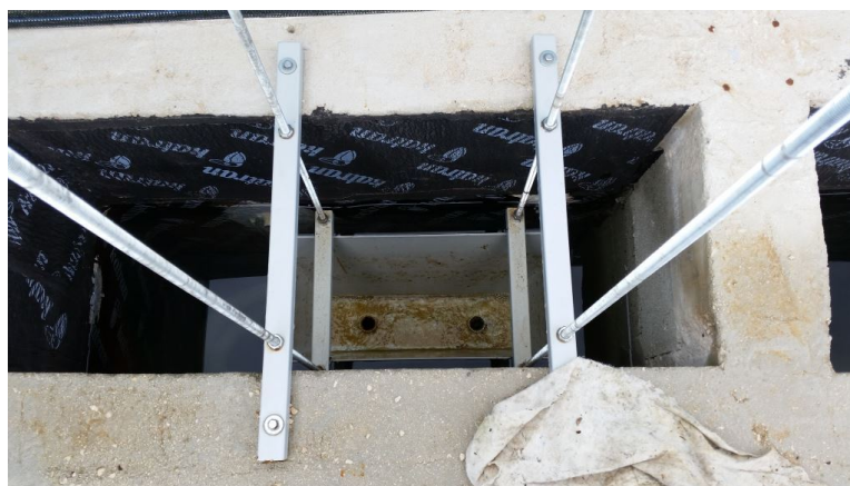
FIGURE A.16: Overflow in upstream reservoir.
