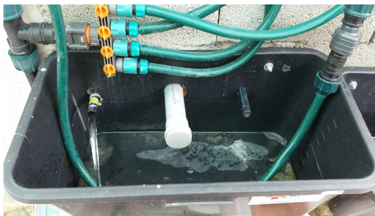
FIGURE A.4: Photography of three conduit outlets.
