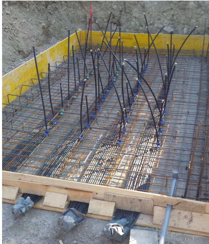
FIGURE A.19: Installation of piezometers.
