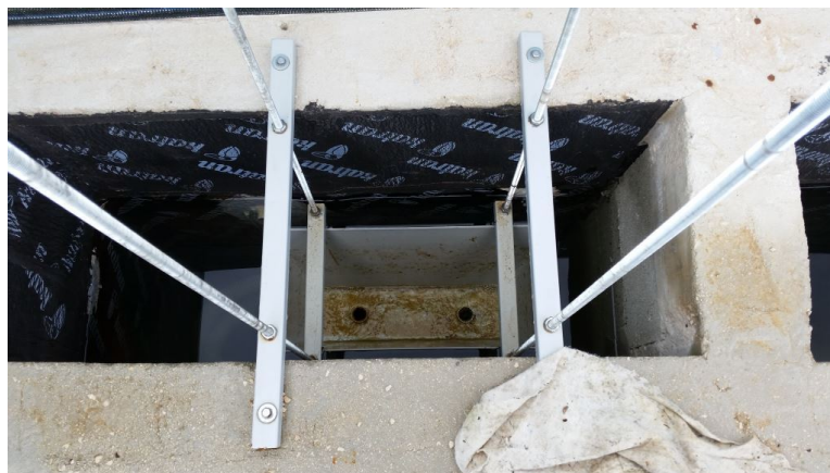
FIGURE A.16: Overflow in upstream reservoir.
