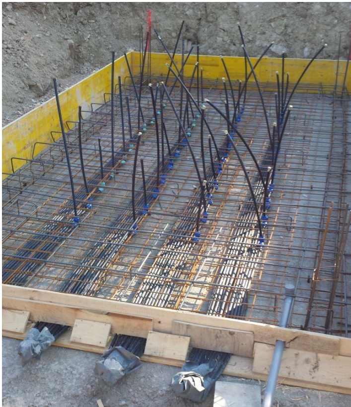
FIGURE A.19: Installation of piezometers.
