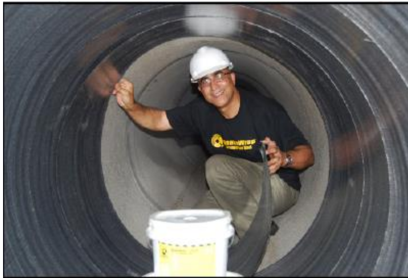
Slika 35. Spiral wound plastic liners [11]
