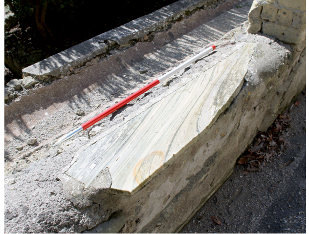
Fig. 19. Herculaneum, House of the Gem, detail of cipollino window sill (photo: S. Barker)
