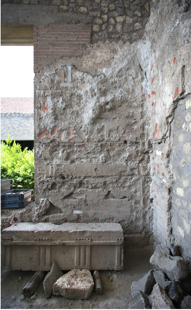
Fig. 18. Pompeii, House of Marcus Fabius Rufus, Room 21, N-W corner, imprint of wall revetment (photo: S. Barker)
