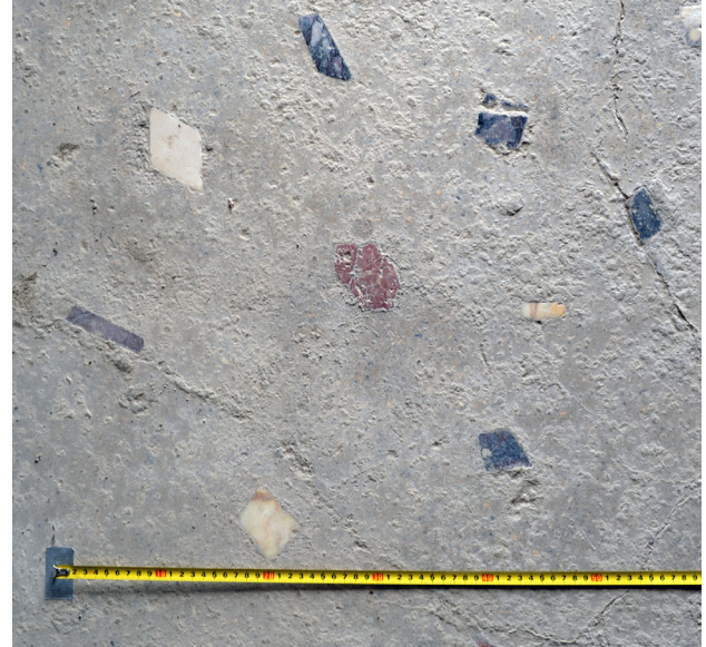
Fig. 4. Stabiae, Villa Arianna, Room M, detail of cement pavement with marble inserts (photo: S. Barker)
