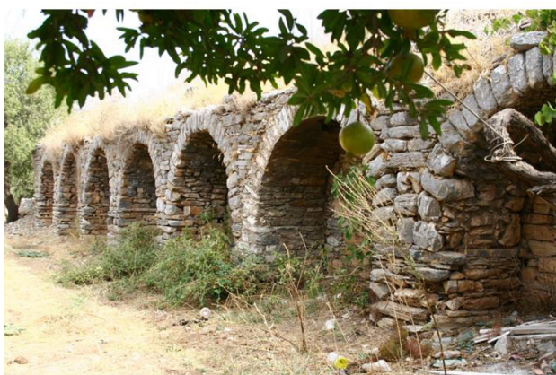
Fig. 9. Above the monumental tomb where marble slabs were sawn; below the nearby aqueduct (photo: M. Molinari)
