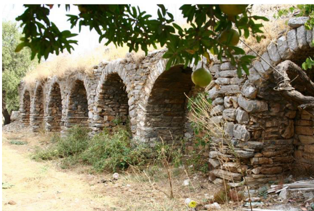
Fig. 9. Above the monumental tomb where marble slabs were sawn; below the nearby aqueduct (photo: M. Molinari)
