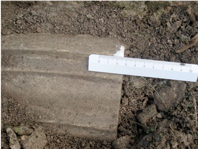
Fig. 5. The curved cornice of a niche
