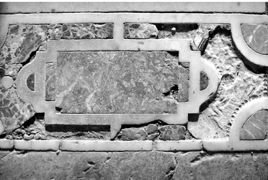
Fig. 8. Example of “inlay” technique; the carved cavity can be seen where one marble slab is missing
