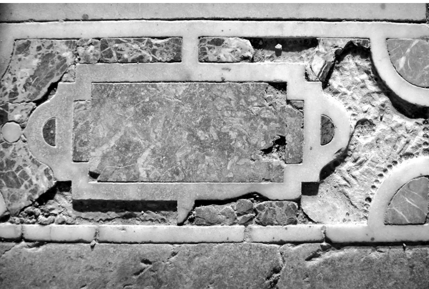
Fig. 8. Example of “inlay” technique; the carved cavity can be seen where one marble slab is missing
