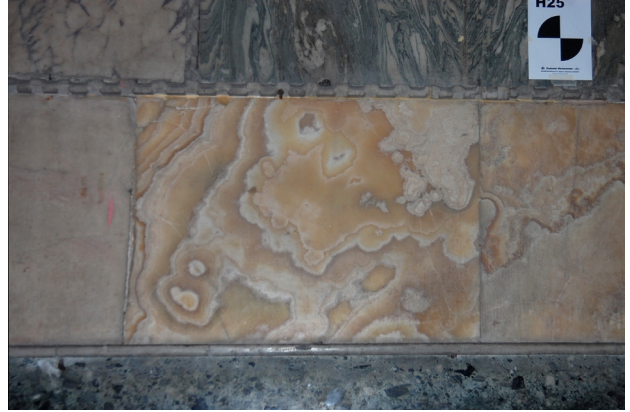
Fig. 3. Hagia Sophia, nave piers, onyx band; at center and right, Egyptian alabaster; at left, white marble?
