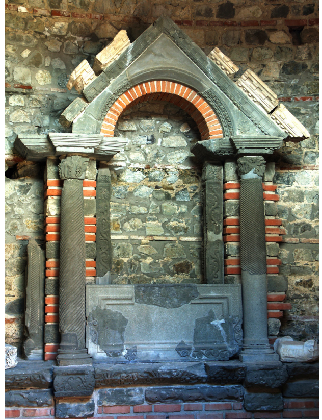
Fig. 5. Architectural elements of volcaniclastic sandstone above the gateways (photo: B. Djurić)
