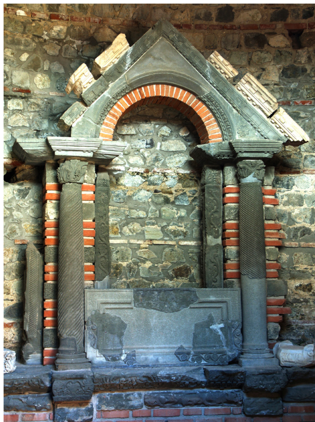
Fig. 5. Architectural elements of volcaniclastic sandstone above the gateways (photo: B. Djurić)
