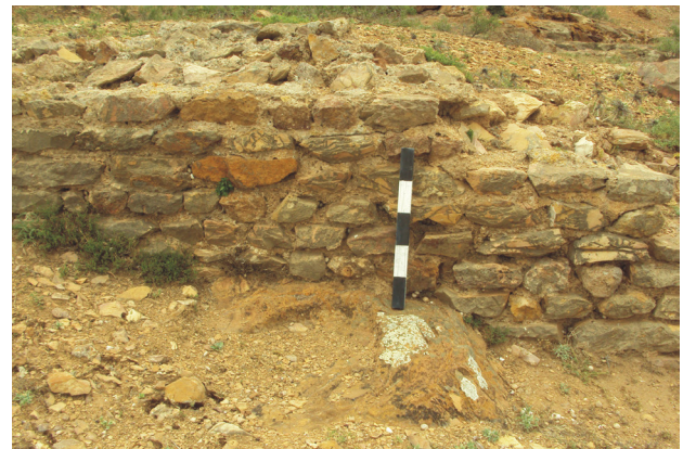
Fig. 11b. Green schist and antique yellow rubble stones used to build construction walls (photo: A. Younès)
