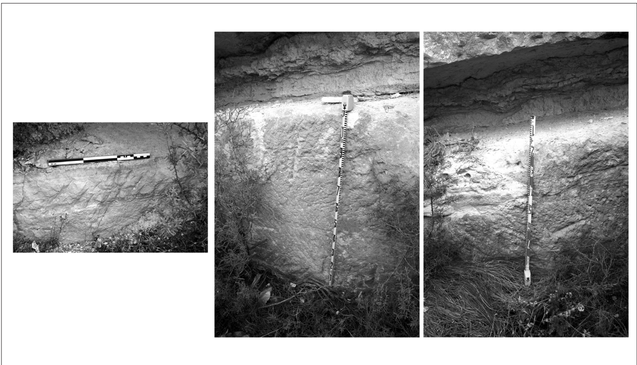
Fig. 4. View of the current state of some of the extraction fronts located on the east slope of the Zahorras River. The marks left by the pick during the block extraction process can still be observed on their surface
